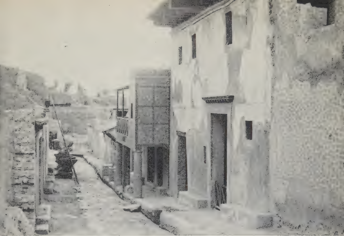
Street in Herculaneum, showing house with balcony and, on the right wall, an example of opus incertum
